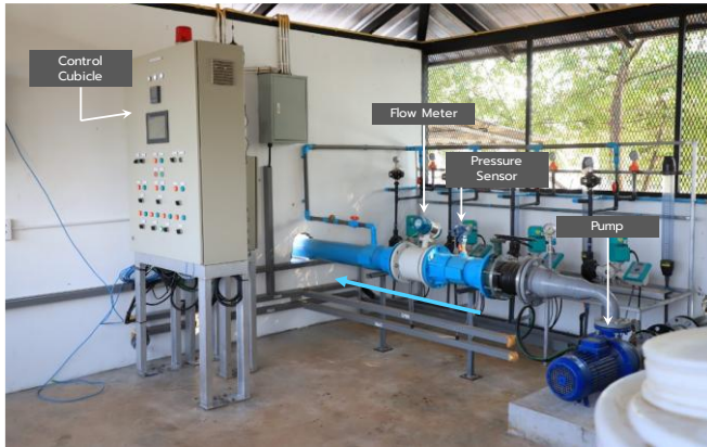
Fig. 9. Pumping Station and Control Panel.
