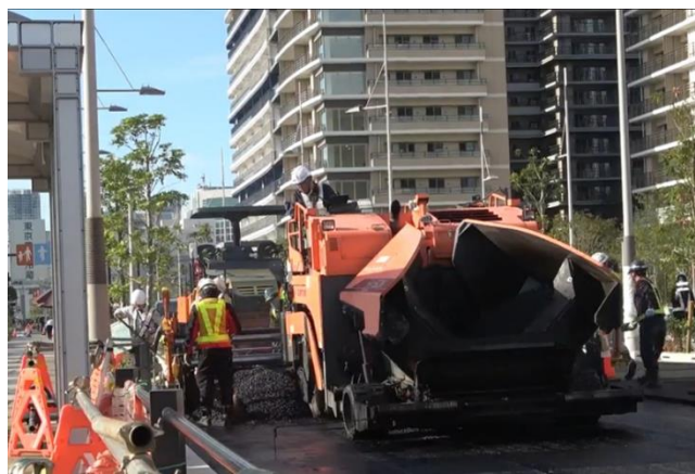
Fig. 17. Eye-level changing with the position of the worker and the resulting forward tilt (paving site in Japan, photo by the authors).
