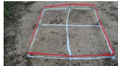
(a) Preparation of test bed
