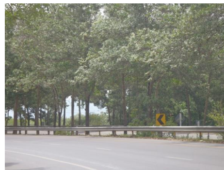
Fig. 3. Guard rails were installed to protect errant vehicles from impacting trees.
