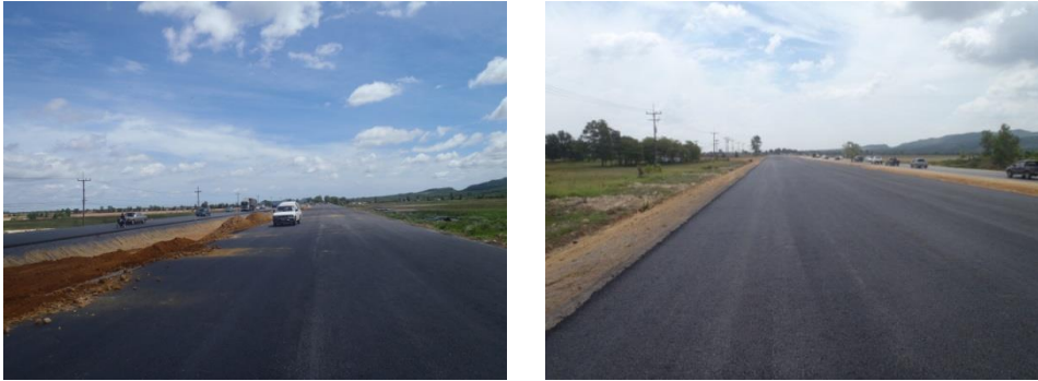
Fig. 5. Improvement in roadside safety after treatment of median by removal of trees.
