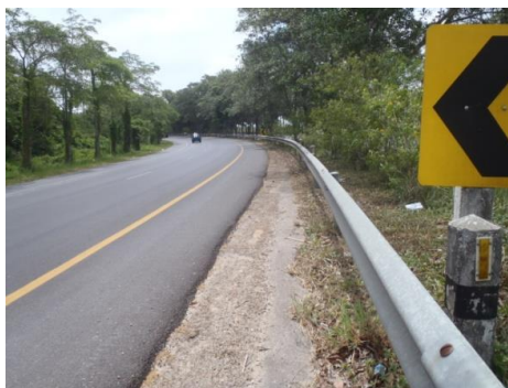
Fig. 3. Guard rails were installed to protect errant vehicles from impacting trees.
