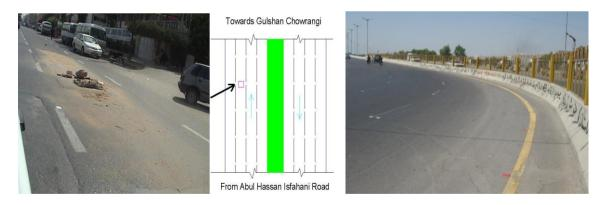
Fig. 1. Open manholes on busy collectors (left) and sharp horizontal curves with no safety measures (right).
