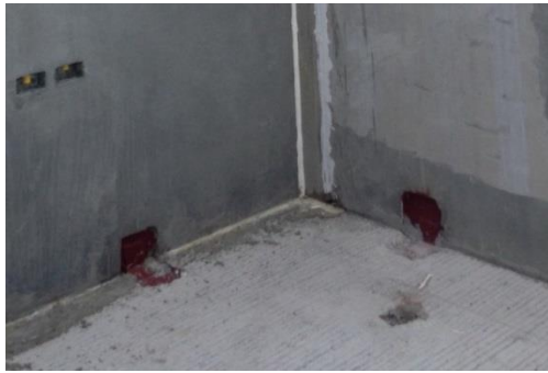
Fig. 6. Connection detail of Welding of steel plate embedded in precast concrete wall and insert plate.
