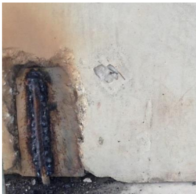
Fig. 7. Connection detail of Welding between dowel bar embedded in lower precast concrete wall and steel plate embedded in upper precast concrete wall.
