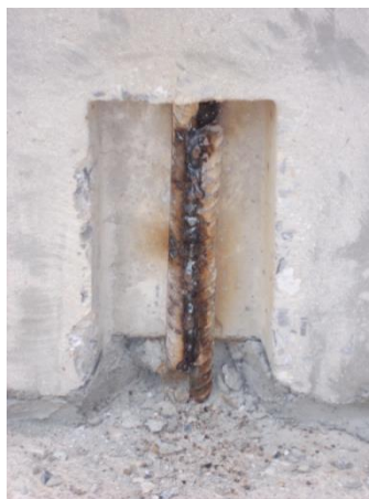
Fig. 5. Connection detail of welding between dowel bars embedded in precast concrete wall.
