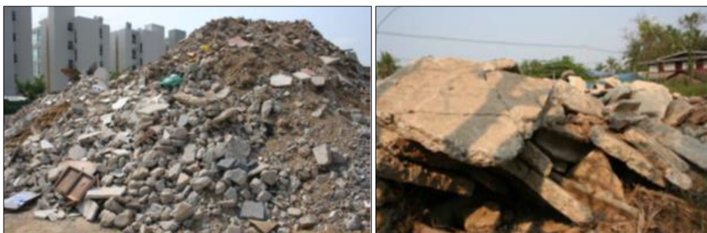
Fig. 2. Demolished concrete in public area of Bangkok [3].
